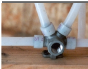
Installation of piping and head manifold during construction
